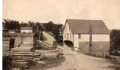
A flood in 1924 gutted the grist mill and carried away the machinery and millstones. Image courtesy of Evelyn Brant.
