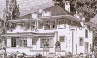
Sears draftsmen added a "Spanish flavor" to the classic American Four-square form and called it "Alhambra" for its California Mission style details. From the Sears Building Materials Catalog, 1924.
