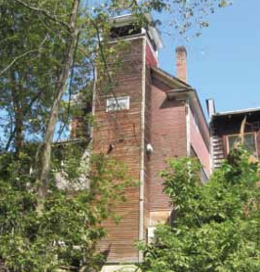
Firemen hung wet hoses in the tower of the "Old Hose House" to dry them after a fire. The bell that hung in an adjacent belfry was moved to the new fire station (1960) on Champlain Avenue. Photograph by Virginia Westbrook.
