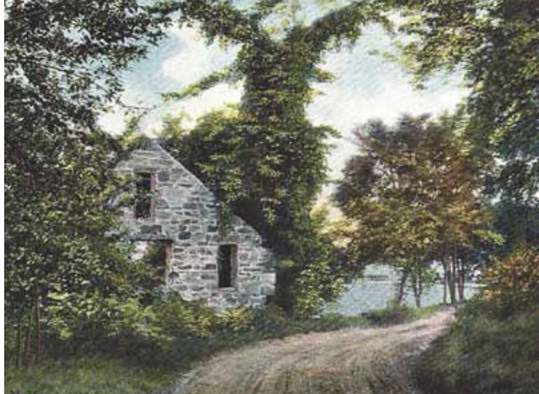
The stone grist mill rose three stories up from its wharf at lake level. The shoreline section of Washington Street, formerly Mill Street, follows the course of James Allen's delivery canal. Photograph courtesy of Bradamant Realty.
