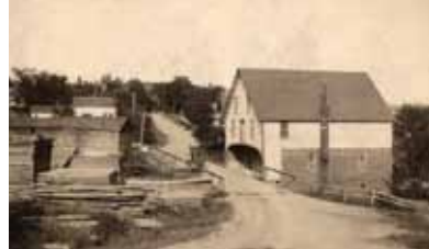
A flood in 1924 gutted the grist mill and carried away the machinery and millstones. Image courtesy of Evelyn Brant.
